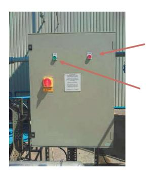
OP1-Push and hold RED button for 2 seconds to close valve(s)
